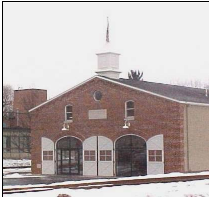
Figure 8: Lewisburg, PA Fire Station. (Courtesy Shubha Shrivastava)
