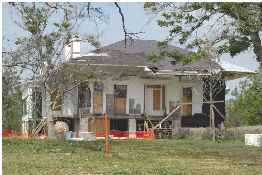
Figure 10: Beauvoir, the National Landmark home of Jefferson Davis, suffered extensive water damage from Hurricane Katrina. Planning to repair the structure and mitigate future damages will involve consideration of the NHPA. (FEMA Photo Library)
