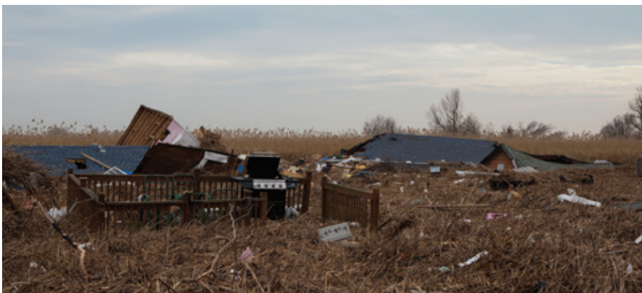
Staten Island, N.Y., Nov. 10, 2012 -- These houses were swept blocks away from where they were built by the flood waters from Hurricane Sandy. FEMA and its state and local partners provided disaster assistance to survivors. FEMA/Tim Burkitt.
