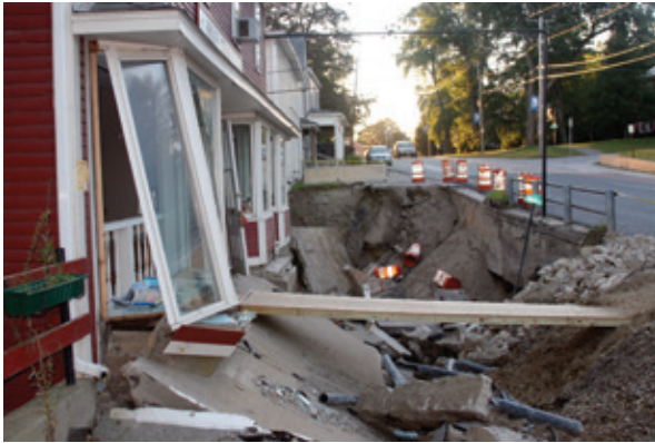
Brandon VT, Vt., September 11, 2011 -- Main Street of Brandon showing damages that Hurricane Irene left behind. Photo by Angela Drexel/FEMA Photo.
