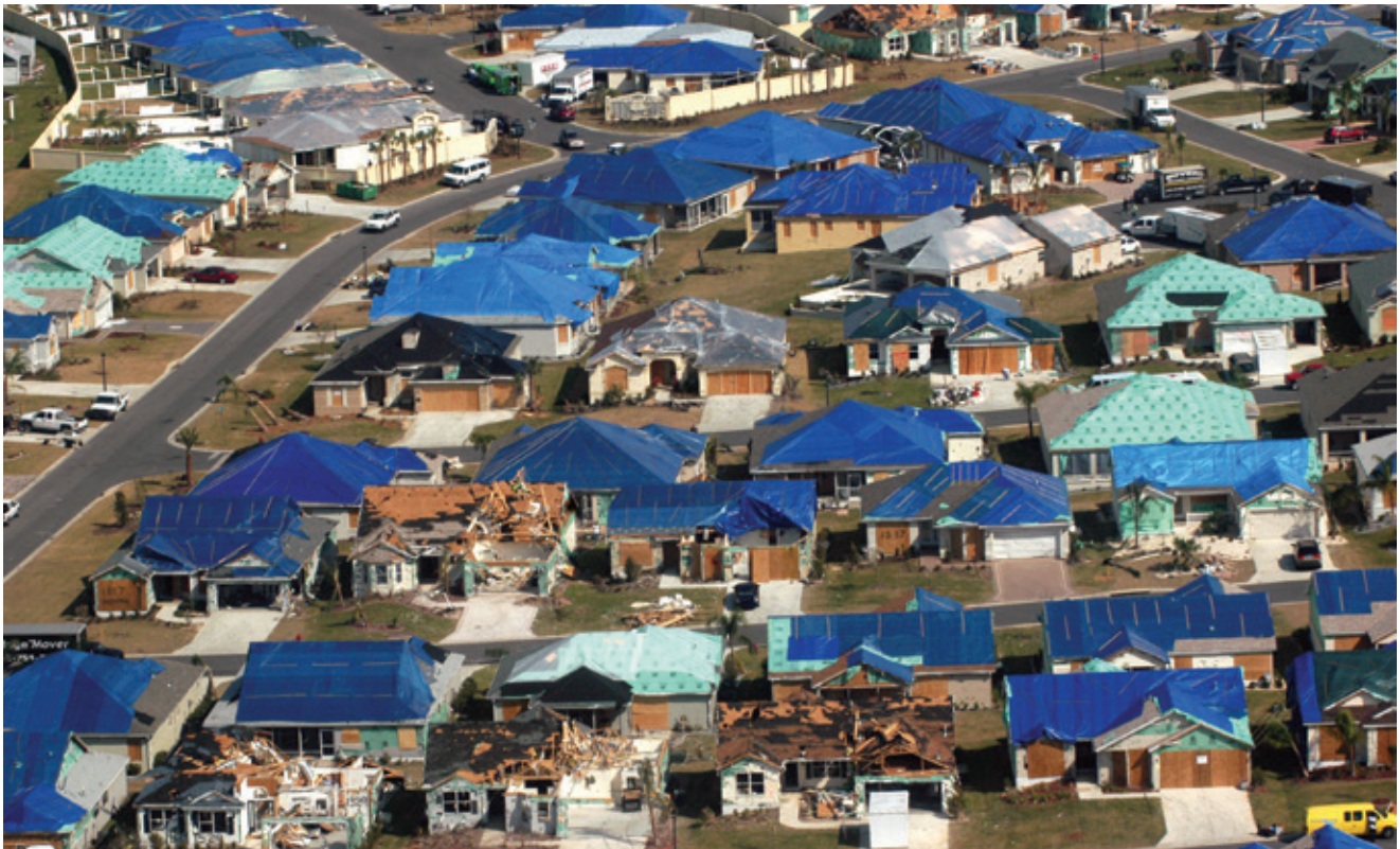
Lake County, Fla., February 3, 2007 -- The damage caused by tornadoes in Central Florida was localized but severe. Mark Wolfe/FEMA.
