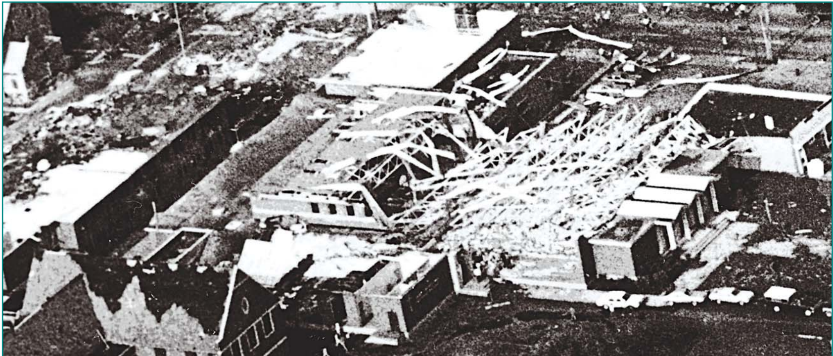
Figure 3-13 St. Augustine Elementary School Gymnasium, Kalamazoo, Michigan.
