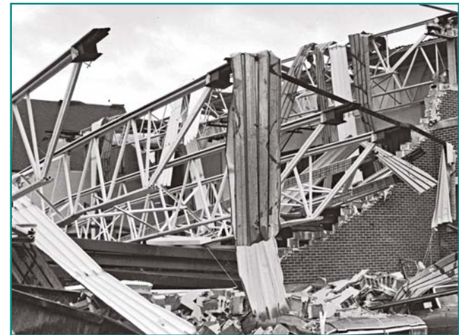
Figure 3-14 Collapsed St. Augustine Elementary School Gymnasium building.
