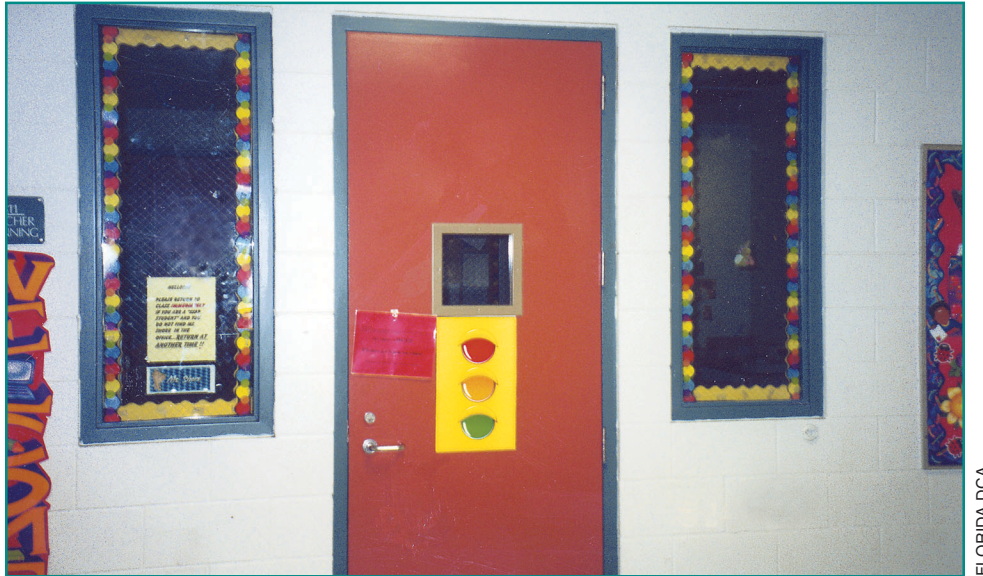
Figure 4-15 Door connecting classroom to corridor – Buildings 200, 400, 600, and 800.
