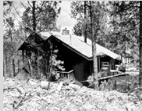
The McDonald home had only minor exterior damage. Homes on both sides were completely destroyed by flames.
