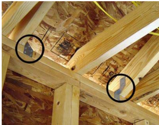
Figure 4: Hurricane clips, shown circled above, help anchor roofs to the main structure to prevent detachment due to severe wind. (FEMA Photo Library)
