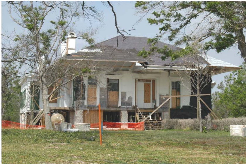
Figure 10: Beauvoir, the National Landmark home of Jefferson Davis, suffered extensive water damage from Hurricane Katrina. Planning to repair the structure and mitigate future damages will involve consideration of the NHPA. (FEMA Photo Library)
