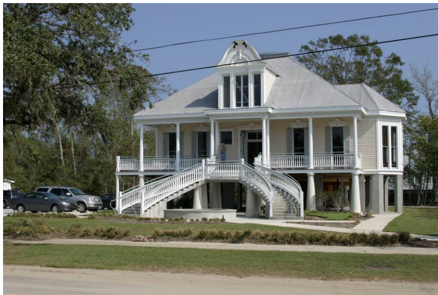
Figure 2: This elevated Louisiana home, which was undamaged by Hurricane Katrina's severe flooding, illustrates one type of mitigation project. (FEMA Photo Library)
