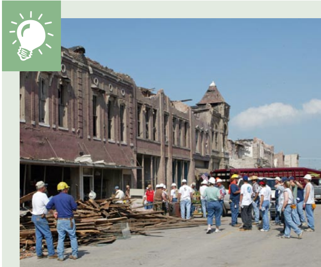
In the wake of a series of tornadoes, many of Pierce City, Missouri's commercial historic buildings were heavily damaged.
