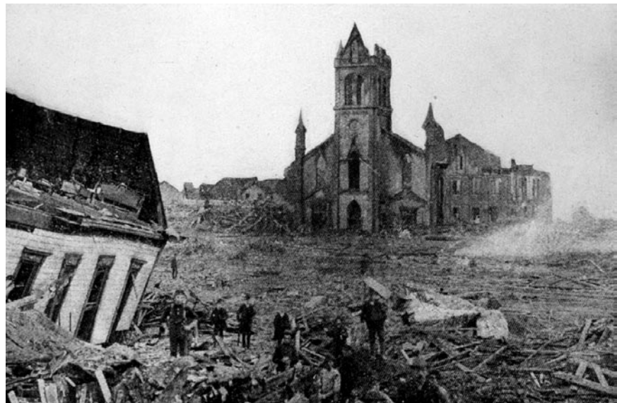
Hurricane and storm surge damage in Galveston, Texas, September 1-10, 1900.
