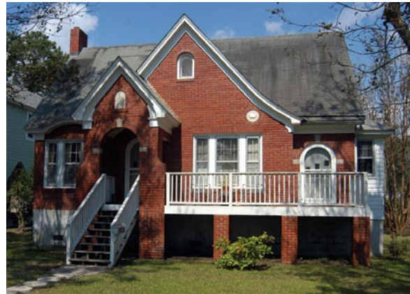
Frame building elevated on concrete block foundation faced with brick veneer. Belhaven, North Carolina.
