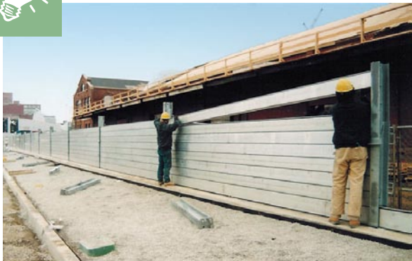
Invisible flood control wall in Louisville, Kentucky.
