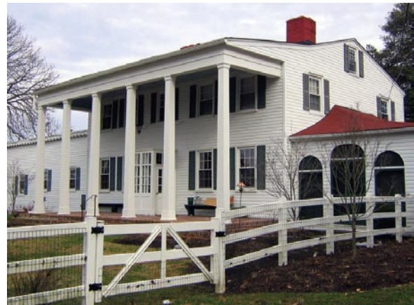
Blythewood has three distinct sections: the 1820s main block (center), 1880s shed-roofed addition (left), and 1920s Colonial Revival addition (right). Prince Georges County, Maryland.
